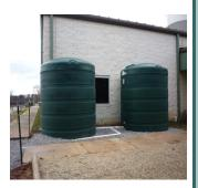
Cisterns up to 5000 gallons can be installed to collect rainwater from buildings and parking lots and be saved for irrigation
